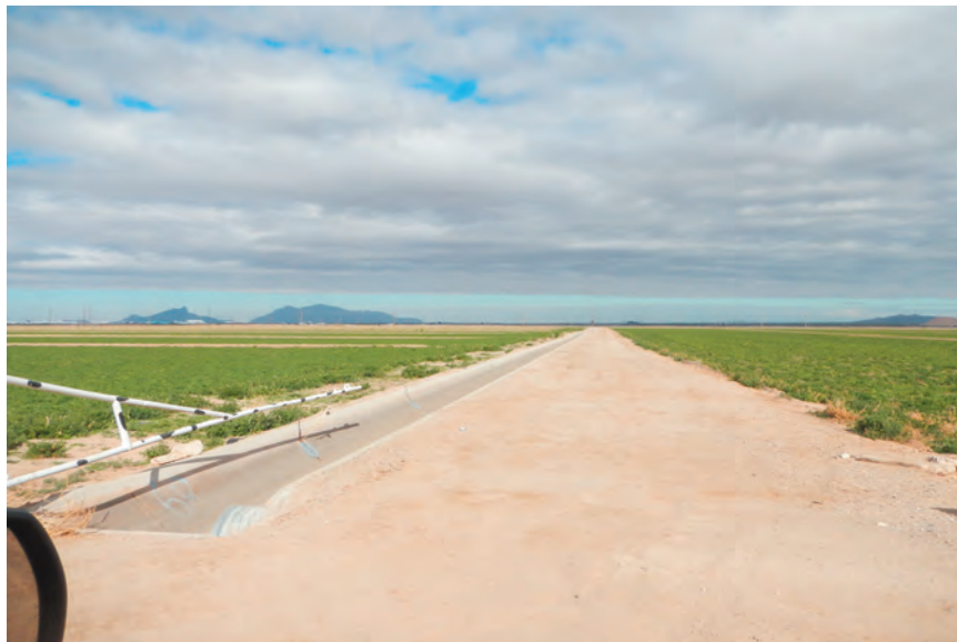
North at Typical Concrete Irrigation Ditch
