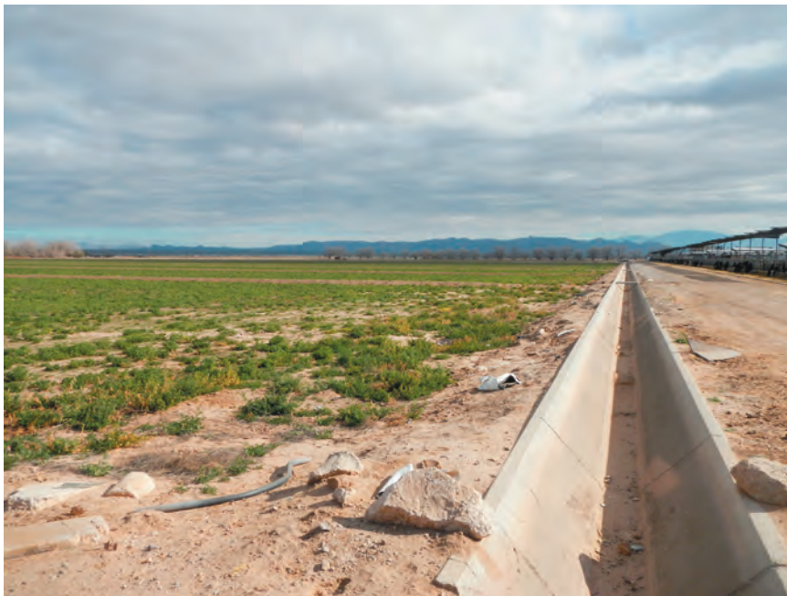
East along Southern Boundary
